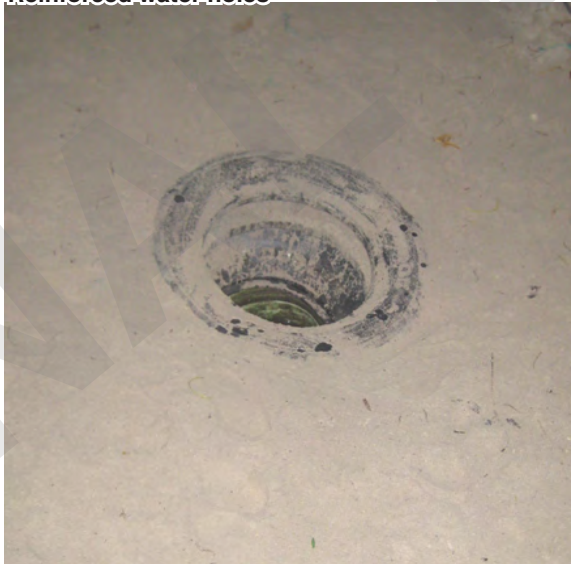
Reinforced water holes
