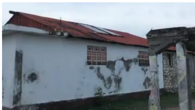
Figure 8: Solar panels installed on roof. 45
